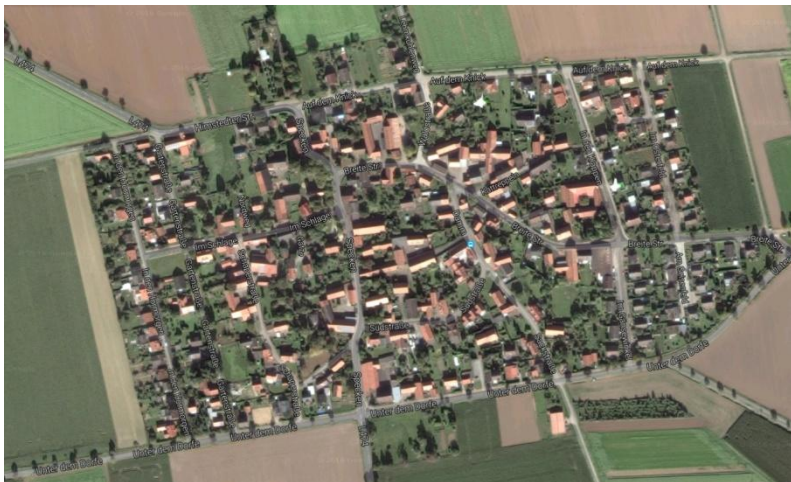
Figure 106. Aerial view of Berel, 2014 (Google satellite photo).
