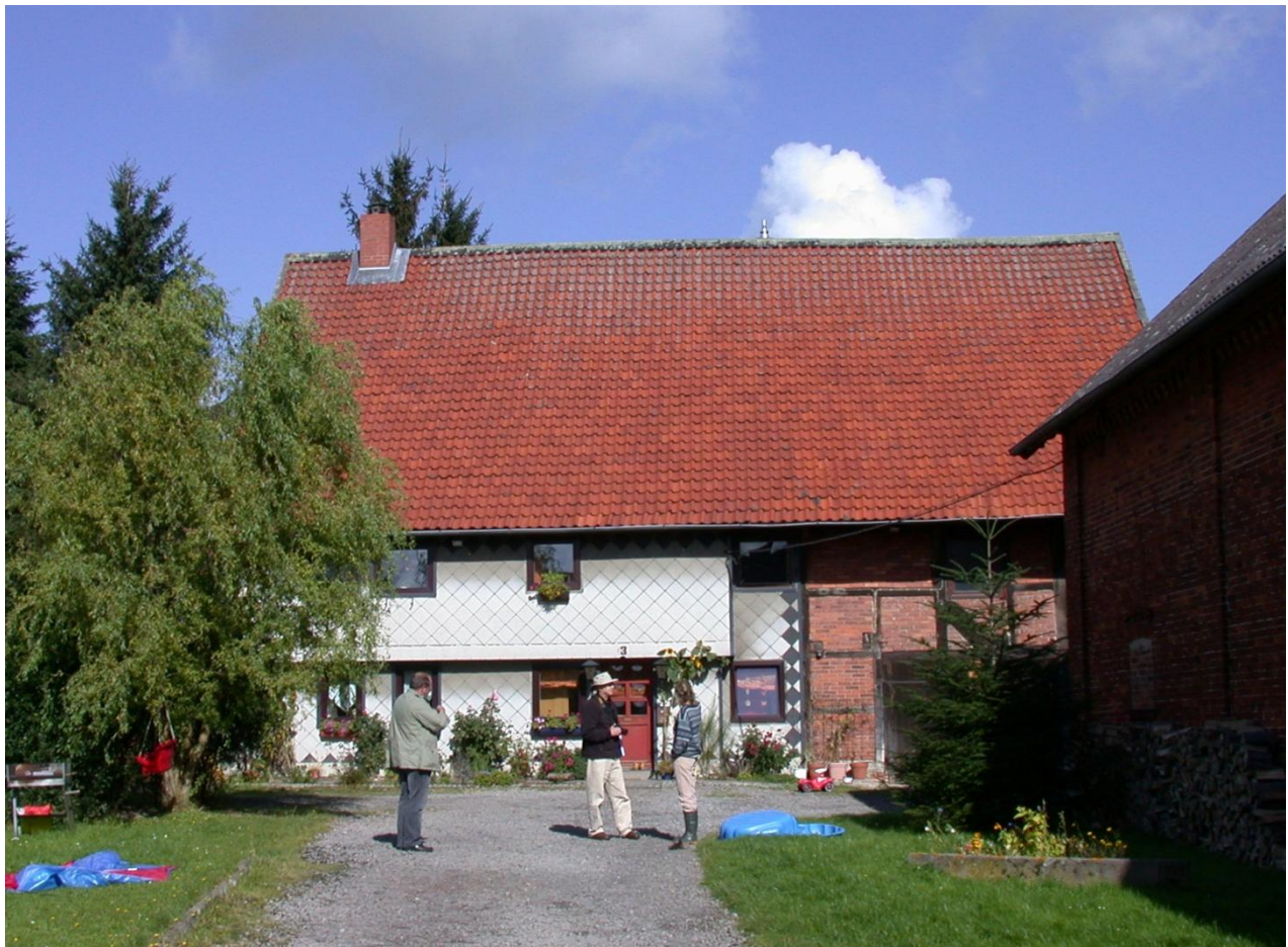
Figure 120. Oldest house in the village of Berel, dating to the 1500s.
